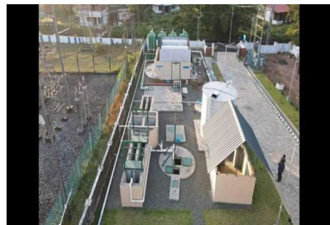
1 MLD CSTP at Padanappalam, Kannur
