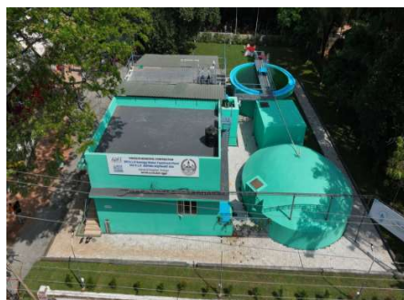
360 KLD STP at General Hospital, Thrissur
